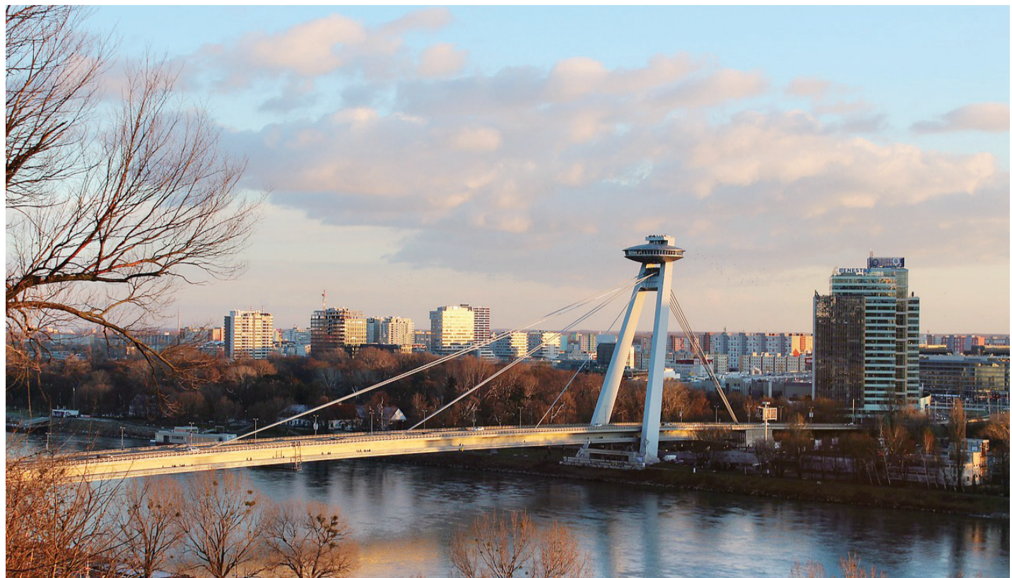
Traversing the Danube, the Bridge of the Slovak National Uprising in the capital Bratislava is among Slovakia's most iconic structures. Called the UFO Bridge by locals, it is the world's longest bridge with one pylon and one cable-stayed plane.
